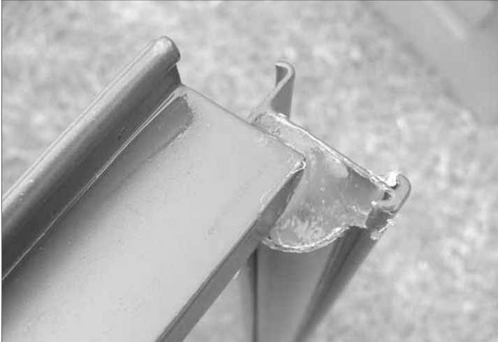
Vent top corner siliconed along with bar capping.
