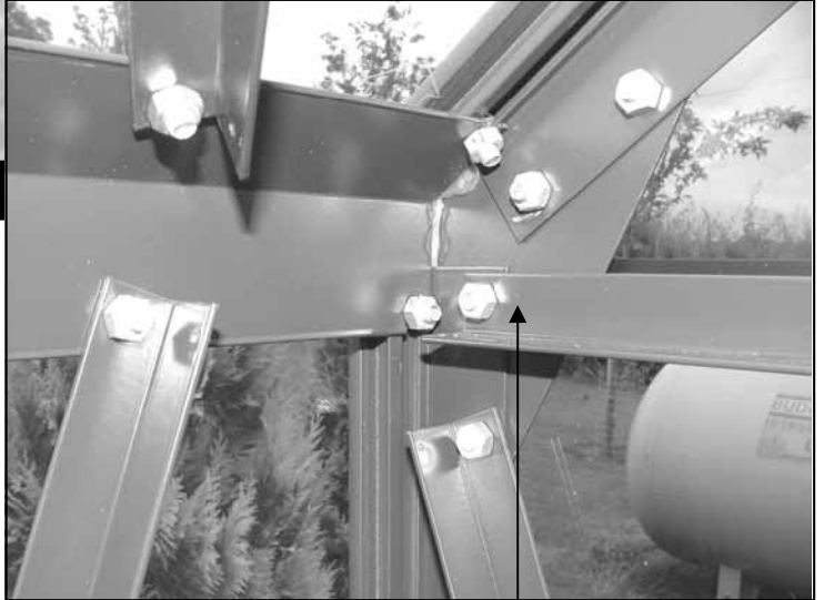
Inside eave area siliconed.
