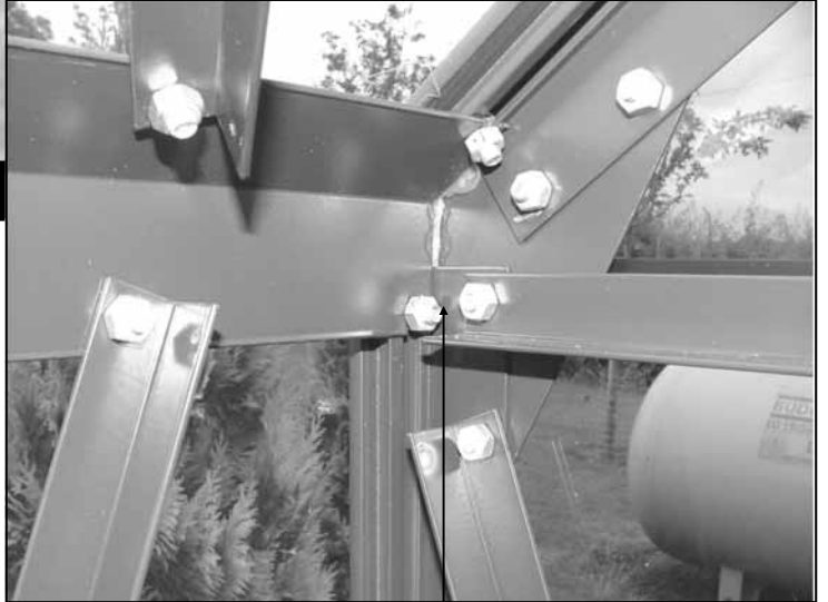
Inside eave area siliconed.
