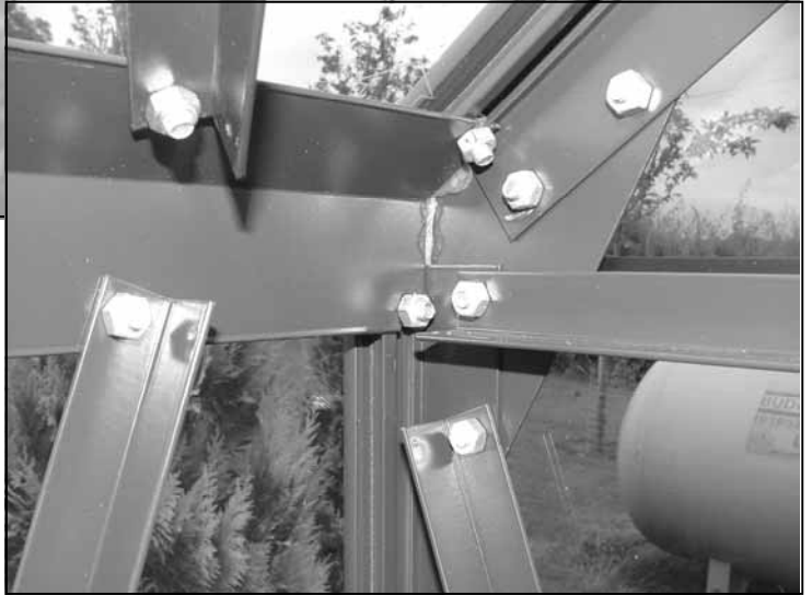
Inside eave area siliconed.
