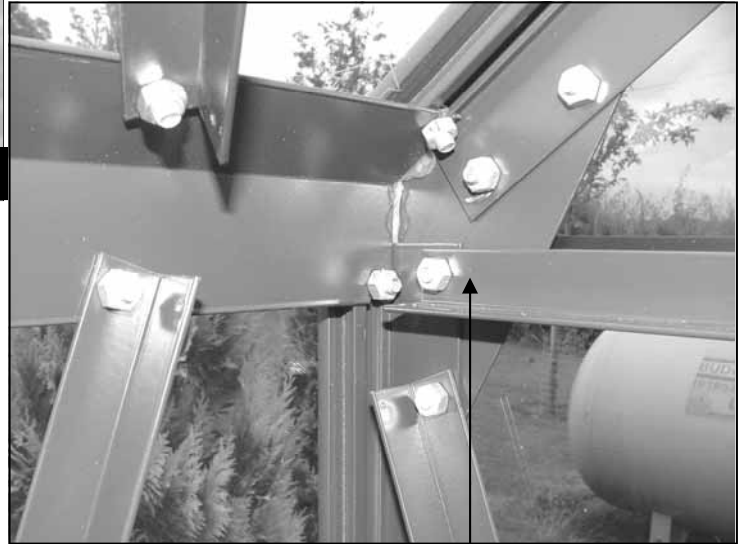
Inside eave area siliconed.
