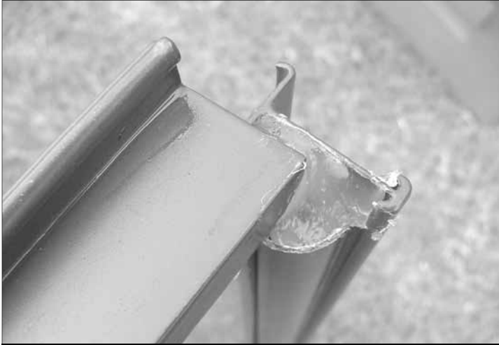
Vent top corner siliconed along with bar capping.
