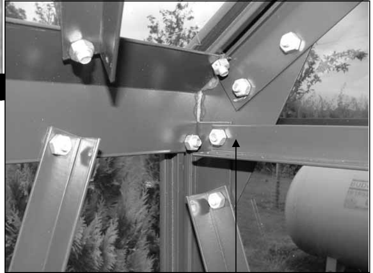
Inside eave area siliconed.
